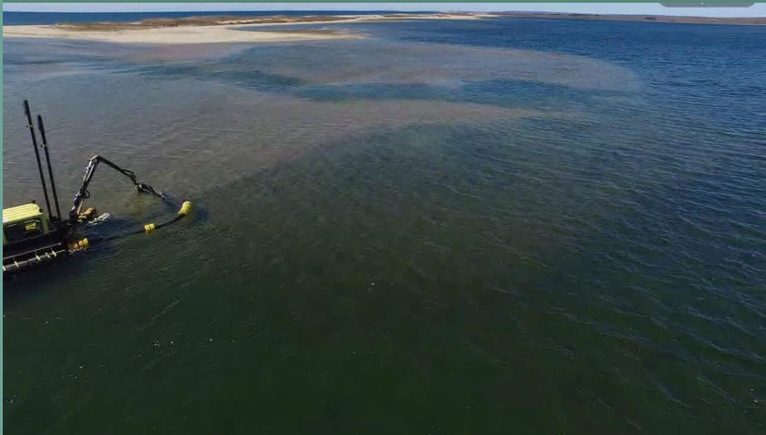
This aerial shot shows “Nessie” beginning to tackle the sandy delta deposited by in-coming water. Above the dredge can be seen a prior channel leading to the new opening of the barrier beach (at very top of the photo).
